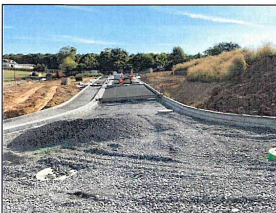
Bsp. Talheim (2020) Bauphase
